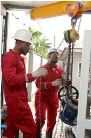
Rigging up a valve with the jig crane
